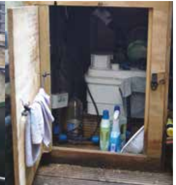
The original Saniflo has its own casing in the dock and takes the waste from two WC's for staff and visitors
