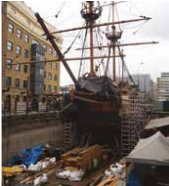
The docks beneath the ship have been turned into a workshop with full joinery equipment
