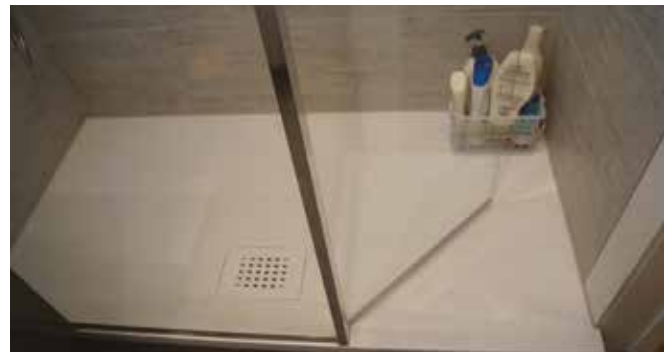
A Kinedo shower tray provides an anti-slip surface as well as low threshold into the shower
