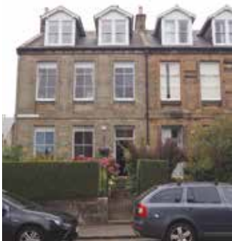
The Victorian Guest House has a plumbing system dating back to the 1800's
