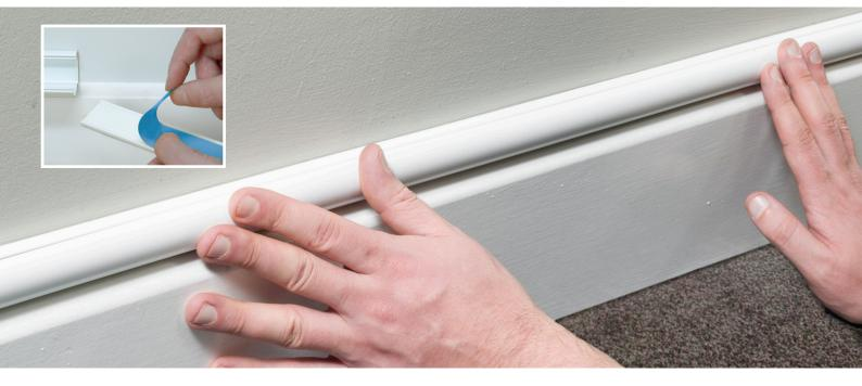
So you've pencil marked the layout of exactly where you want your D-Line cable hider, cut the lengths to size with a fine saw-blade, and considered gaps for any corners or bend accessories to be inserted...
