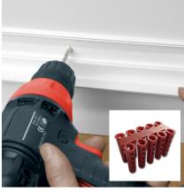
A plasterboard wall should use wall plugs, so the screw attaches through the trunking drill-hole into the wall plug. Screws (& wall plugs) in the trunking should be spaced no more than one metre apart.
