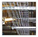
A comprehensive range of stainless steel cable basket and accessories for use in areas where hygiene regulations and tolerance to corrosion require the highest quality products manufactured from the highest quality materials.
