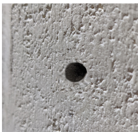
1. Drill a hole
