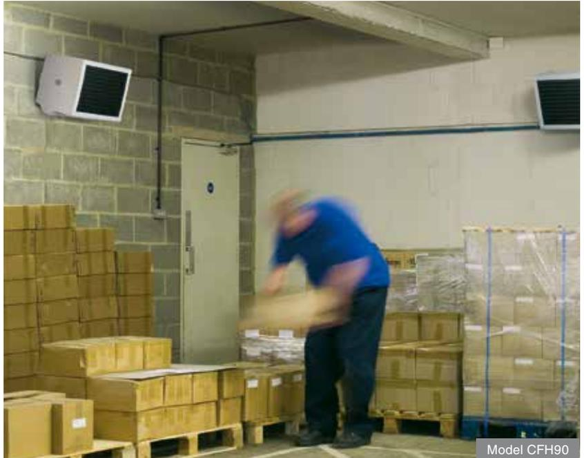
A range of rugged, high-power electronic fan heaters designed to offer a full heating system to larger industrial environments, these wall-mounted heaters use powerful centrifugal blowers for a faster airflow in the most challenging of environments.
