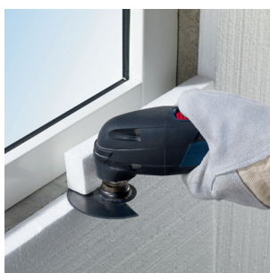
Flush cutting protruding insulation material, e.g. polystyrene
