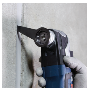
Cutting expansion joints
