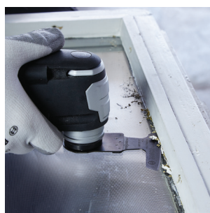
Cutting window putty (sealing compound)
