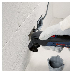
Routing grooves in porous concrete, for laying concealed cables and pipes
