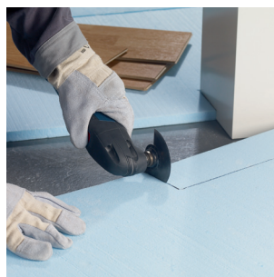
Cutting sound dampening panels, rubber mats, carpet, etc. to size cleanly and efficiently
