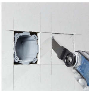
Problem-free plunge cuts in plasterboard
