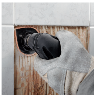
Removing stubborn mortar or tile adhesive, e.g. when replacing damaged tiles
