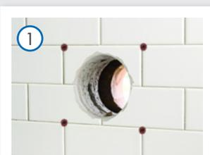
1 Remove the old fan and its wiring from the wall or ceiling.
