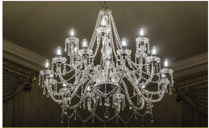
Integral LED filament lamps are installed in over 30 chandeliers at Wollaton Hall, Nottingham.
